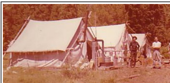
Lochsa Highway 12 construction crews bunk in two tents at Post Office Creek, take meals in third tent.
